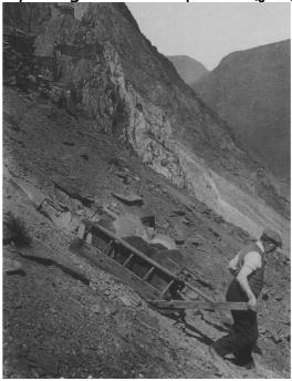
• In the 1880s railway tracks carried trucks of slate. These were controlled by cables from a drumhouse. These were called self-acting inclines, as the weight went up, the truck went down with slate in it, and when the weight went down the truck went back up for more slate.
